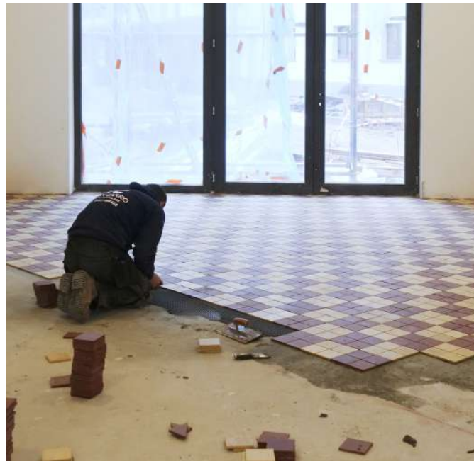
Illustration of the general principles of reuse through the case of a tiled floor: careful dismantling, transport, cleaning and reuse.
