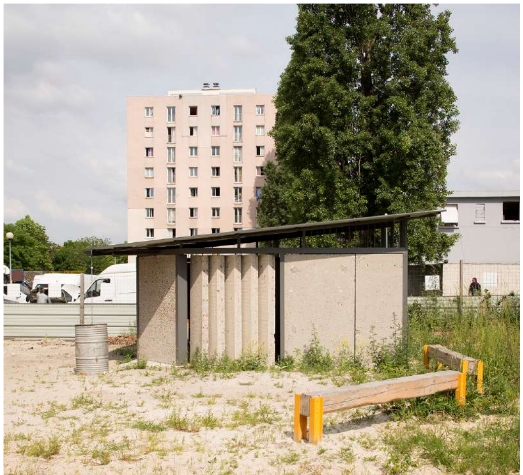
La Fabrique du Clos in Stains, deployment of the concrete reuse sector in a NPNRU project.
